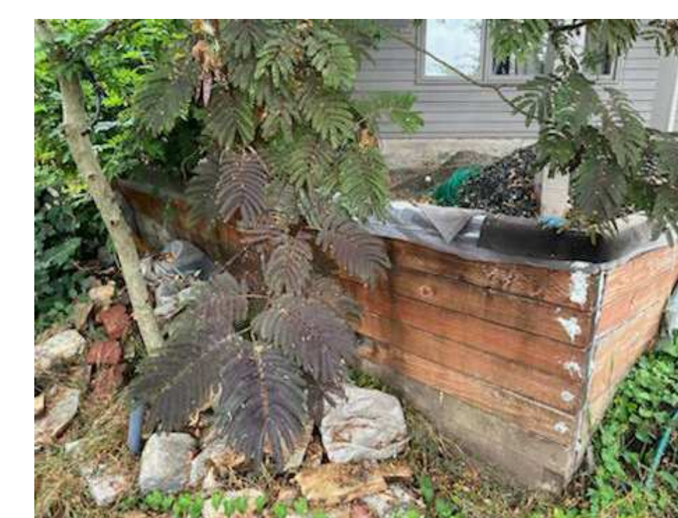
WOOD RETAINING WALL
