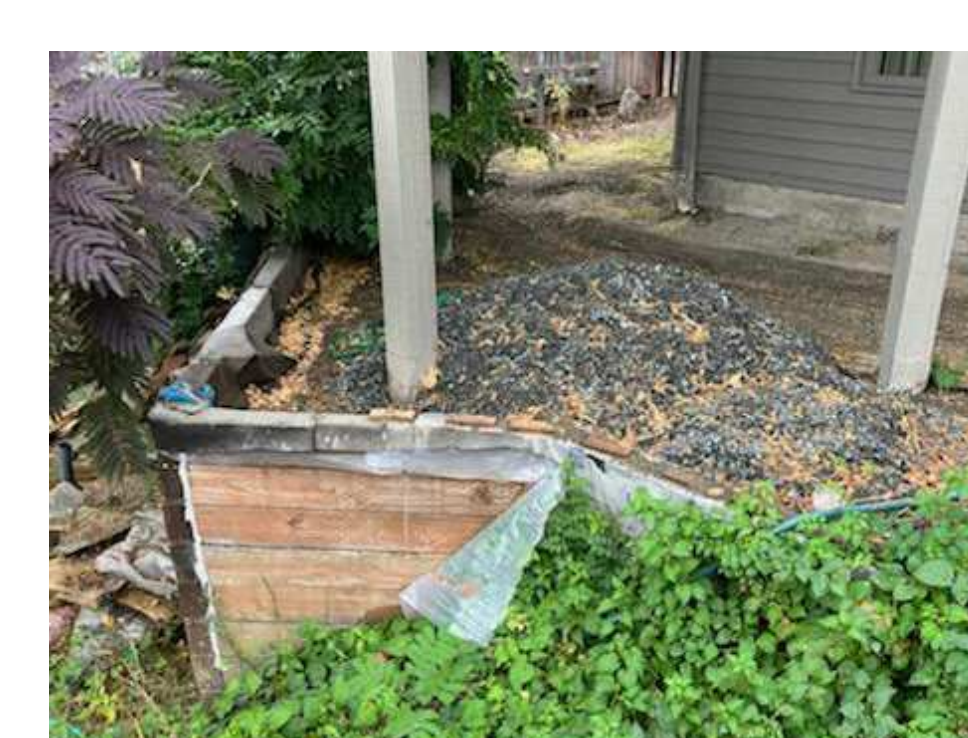
WOOD RETAINING WALL
