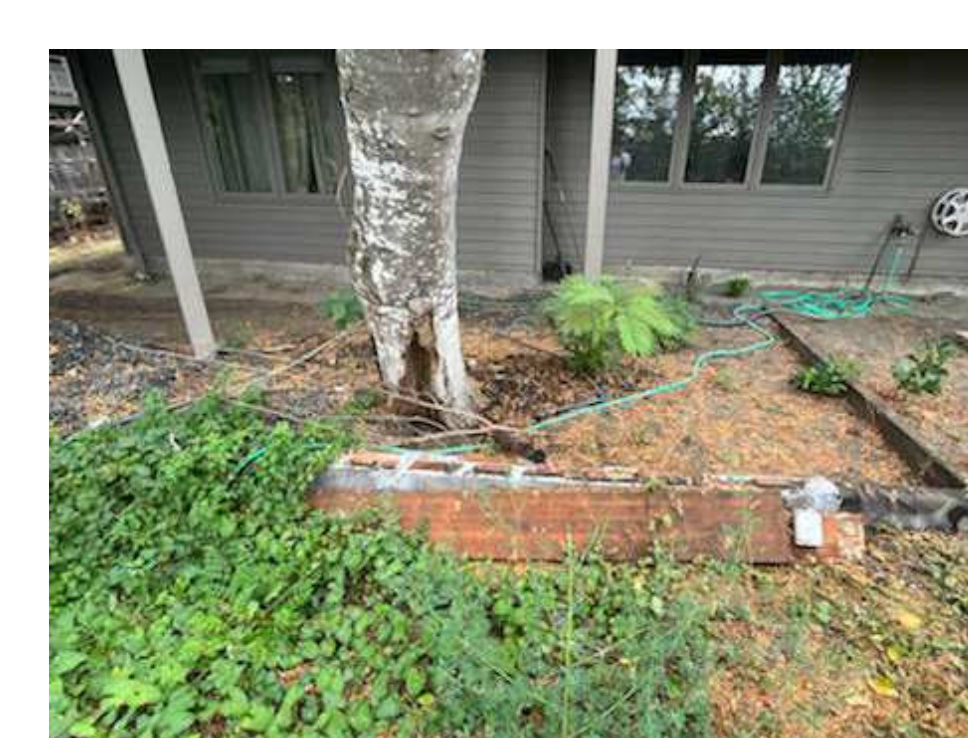
WOOD RETAINING WALL
